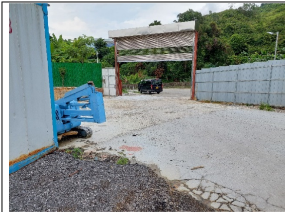
Plate 1 – Existing entrance of the subject site
