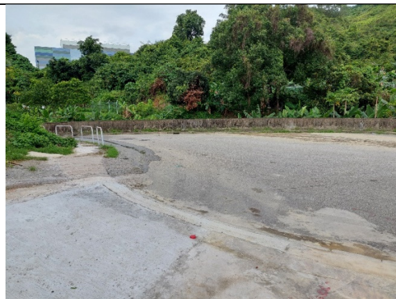
Plate 5 – Existing cul-de-sac of Kam Ho Road in front of the existing entrance of the subject site
